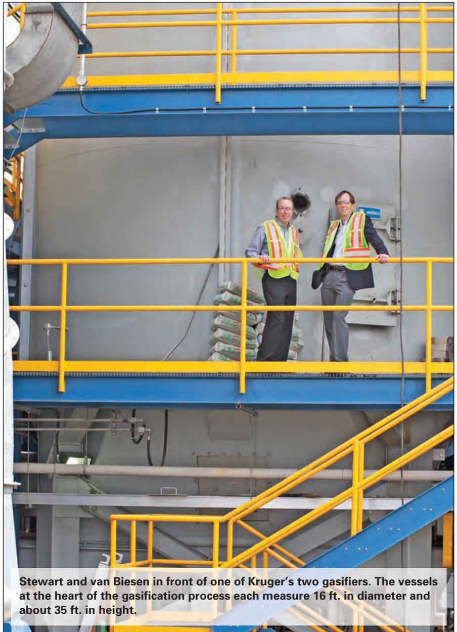
Stewart and van Biesen in front of one of Kruger's two gasifiers. The vessels at the heart of the gasification process each measure 16 ft. in diameter and about 35 ft. in height.
