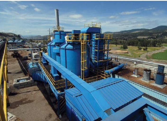
***The syngas produced at the gasification system at Tolko's Heffley Creek operation is burned to generate 40 gigajoules per hour of heat. It will displace about 235,000 gigajoules per year of natural gas that the mill previously used to heat water for log conditioning and veneer drying.***
