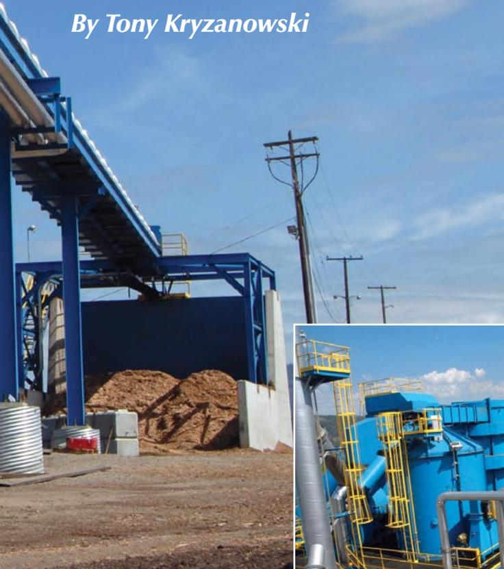
power generation. It is a starved air process that uses heat to convert carbon-containing fuel into syngas.
