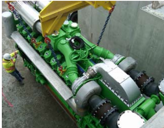
Installing GE Jenbacher Engine at UBC
