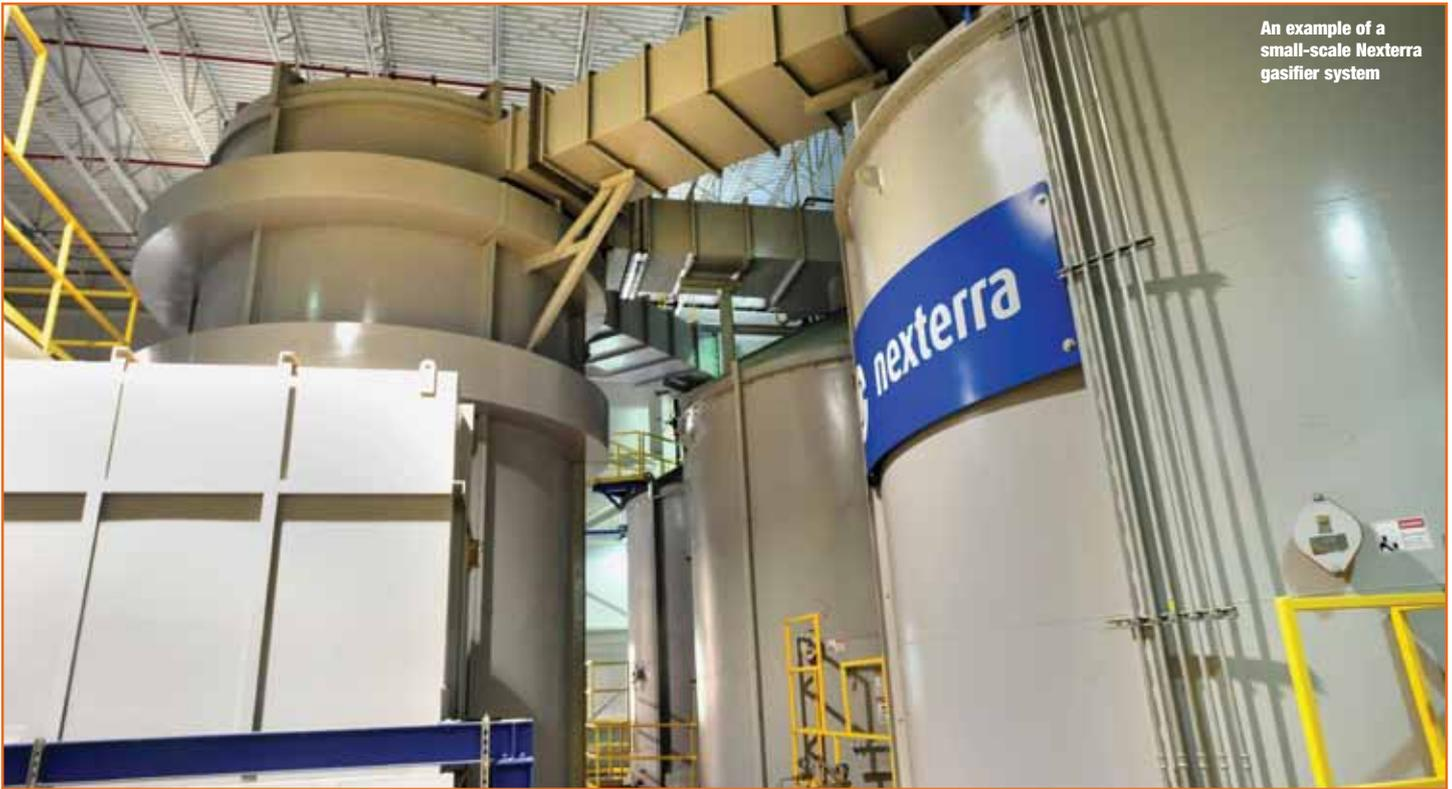
An example of a small-scale Nexterra gasifier system
