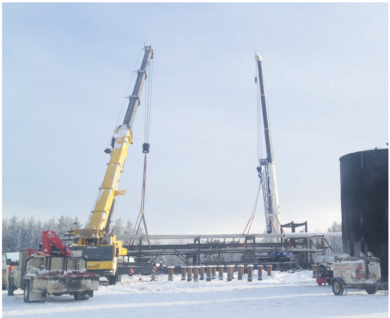
Construction of the N-Solv pilot plant on Suncor's Dover Lease. Companies like N-Solv are helping Canada's oil sands operators protect the environment and perform more efficiently. SUPPLIED
