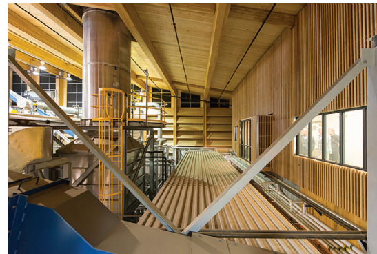
UBC plant under construction
