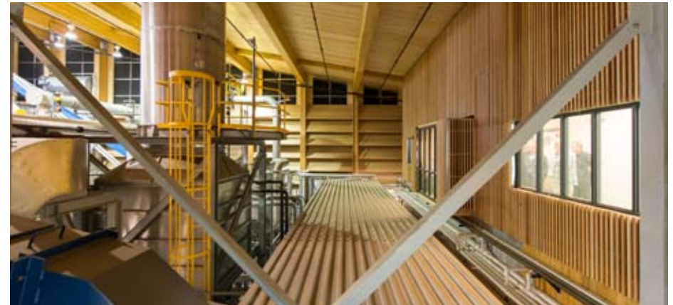
Photos: McFarland Marceau Architects
